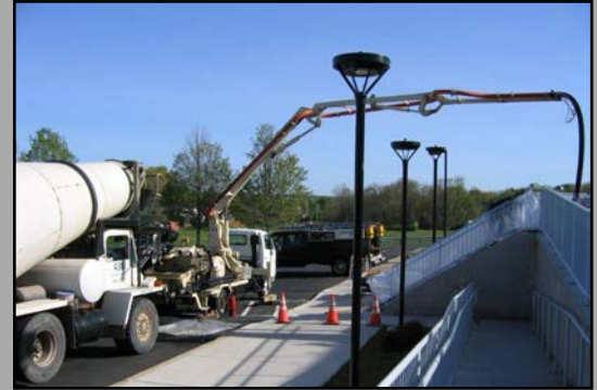
Sidewalks, curbing, dumpster/dolly pads, staircases, ramps, pipe bollards, ADA Compliant solutions
