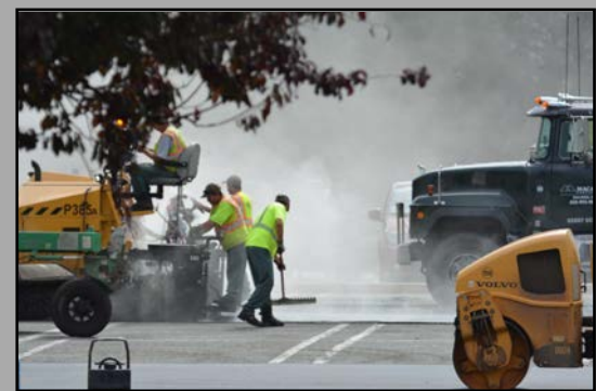
Partial- and full-depth repairs, potholes, sub base excavation and fabric stabilization
