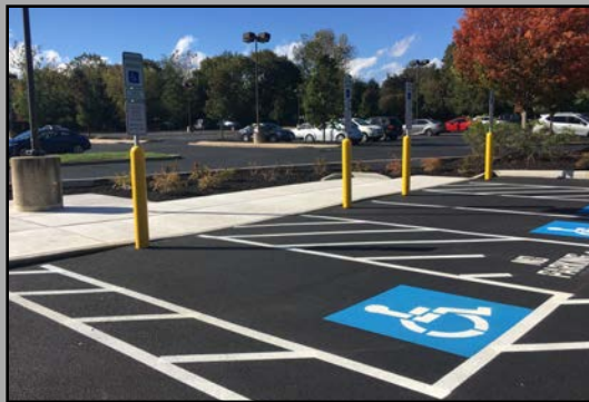
Parking stalls, roadway markings, stenciling, signage, ADA compliant solutions
